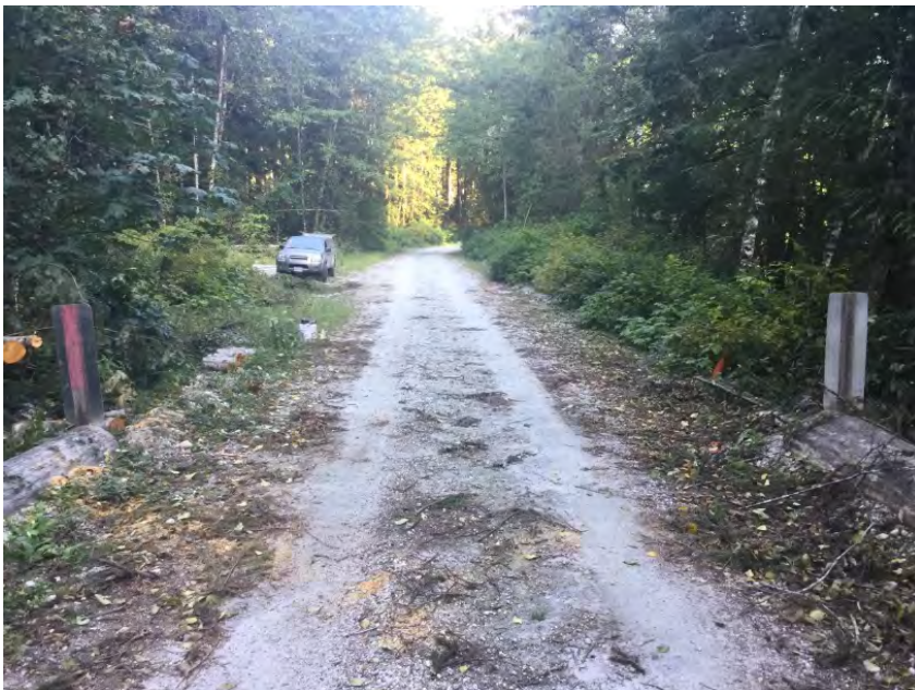
Left Approach Facing Away From Bridge
