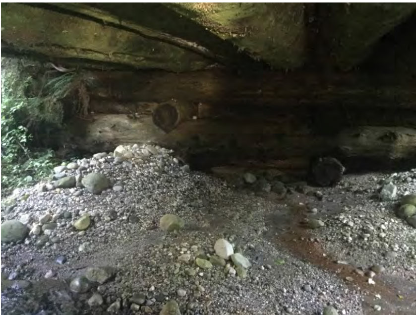
Left Bank Abutment
