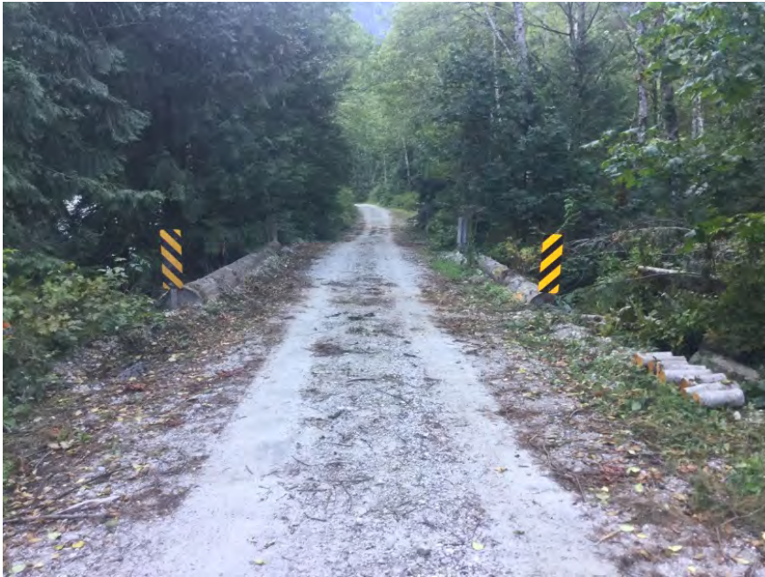
Left Approach Facing Bridge
