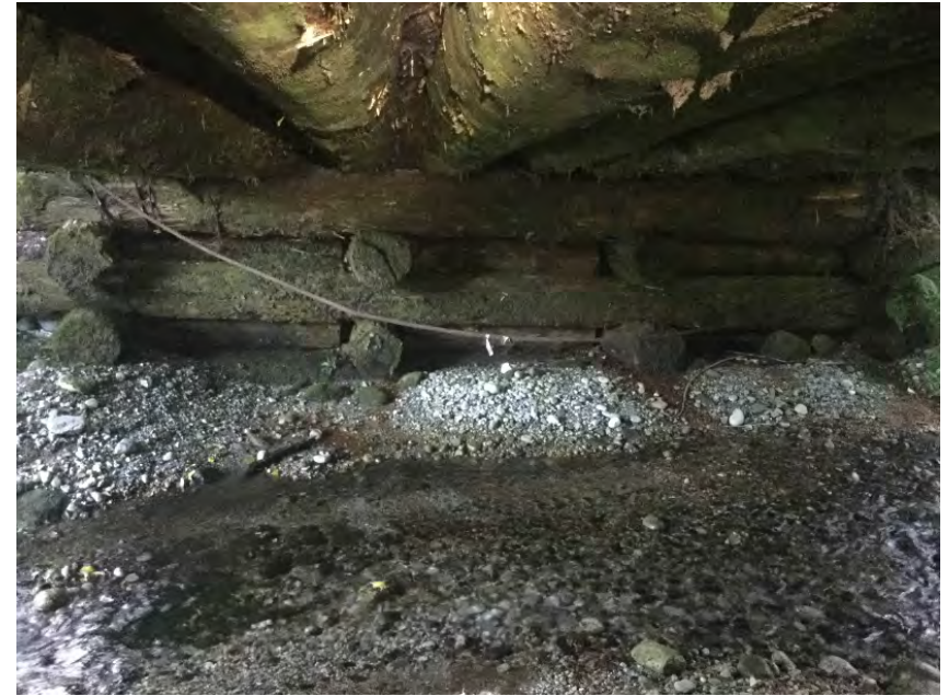
Right Bank Abutment
