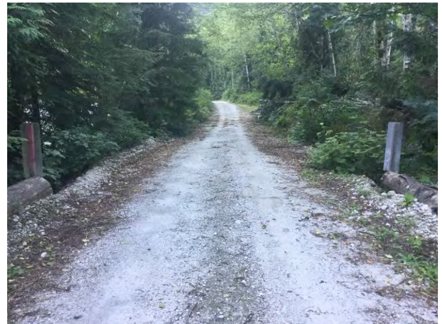
Right Approach Facing Away From Bridge
