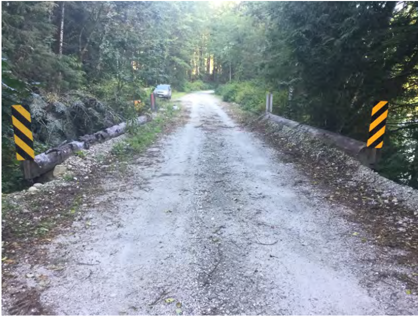
Right Approach Facing Bridge
